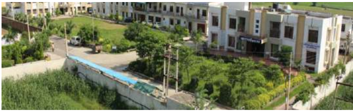
Apna Ghar Ashram (Residential Homes) for helpless destitute persons
