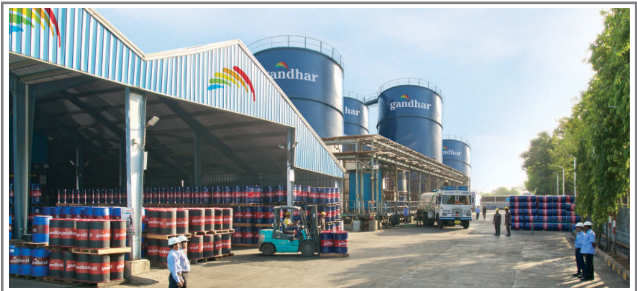
Storage tanks and drums at warehousing facility
